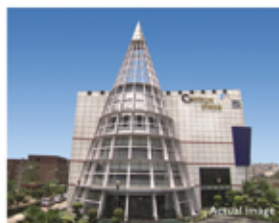
CENTRUM PLAZA, GURGAON Premium Office Complex
